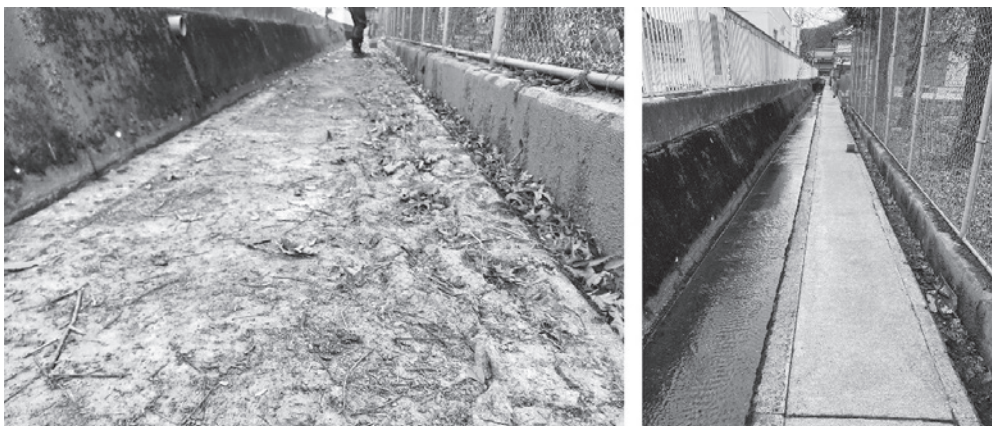
Fig.6 Left: A passageway before cleanup work Right: After cleanup work
