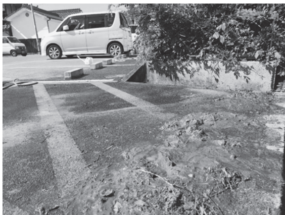
Fig.2 The disaster-affected area at Day Care Center B
